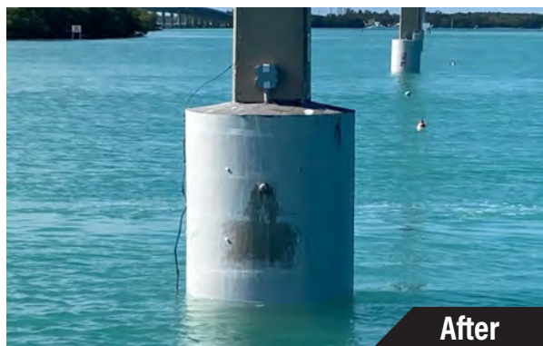
Following the treatment, the transmission pole shows no visible signs of corrosion or concrete spalling.
