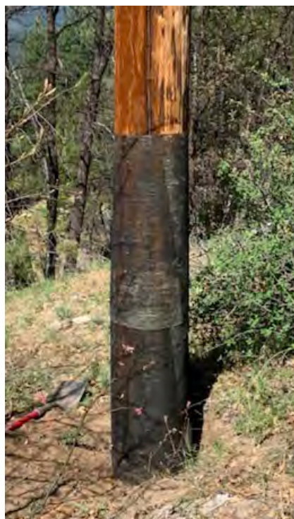
PSREC relies on fire mesh to mitigate fire spread.
