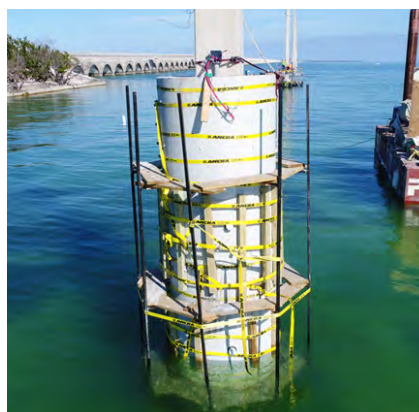
The LifeJacket technology consists of two 50-pound zinc anodes and newly poured concrete.
