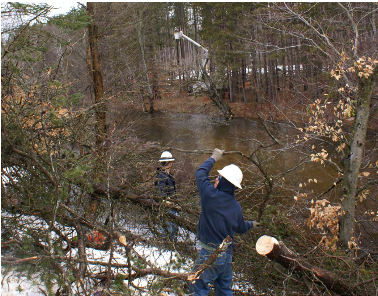
CEC linemen clear tree debris and prepare to pull conductors up from a river bed, while a bucket truck is used to reach a damaged overhead line.
