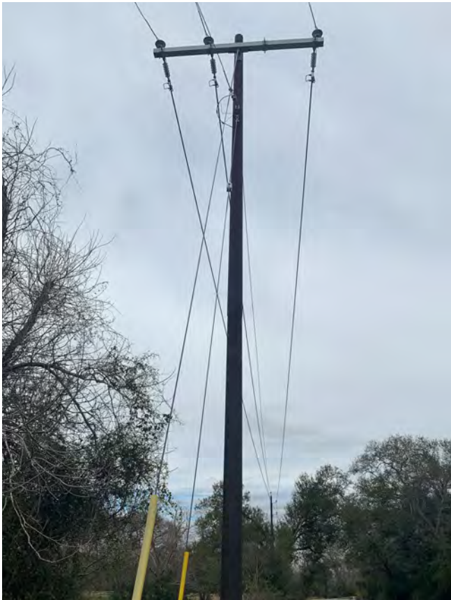
JEC uses direct, burial steel poles in locations that need extra support.
